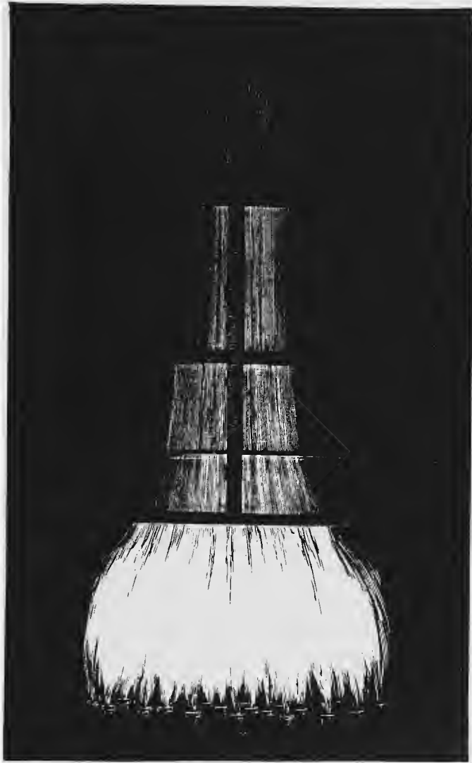
THE IRISH GAS LIGHT FOR LIGHT-HOUSES—108 Jets.
